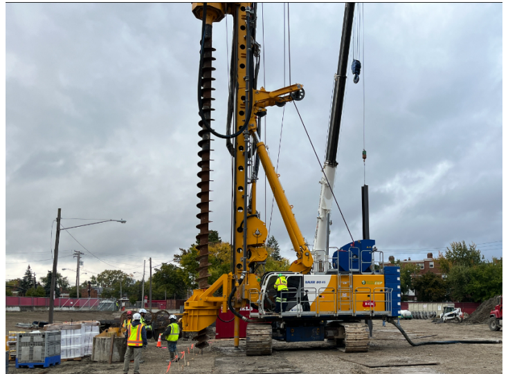
Van Aken District Phase Two Three-Month Construction Look Ahead
