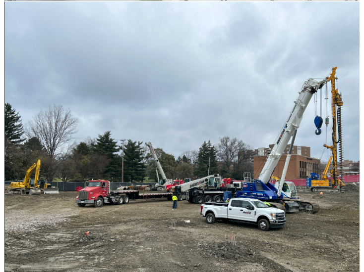
Three-Month Construction Look Ahead
